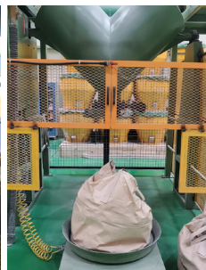
① Safety Fence for Rotating Machinery
