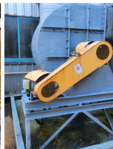
① Safety Cover for Rotating Machinery
